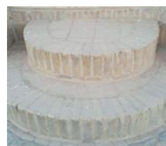
Fig 3 Semi-circle brick stairs
